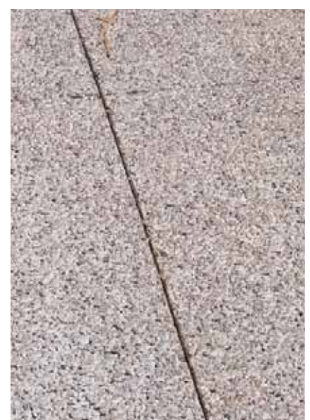
Sawed control joints were installed after the curing operation concluded.
