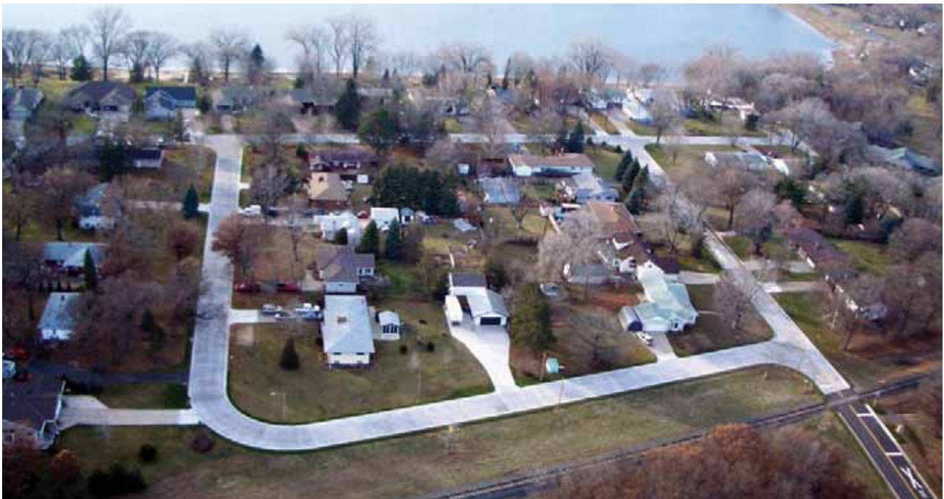
The large, white square stretch of pervious concrete pavement alongside Lake Owasso in Shoreview, Minn., was installed in 2009. At 79,800 sq. ft. and 7 in. thick, it's the largest pervious public street in the U.S. PHOTO: WILLIAM RANDLE
