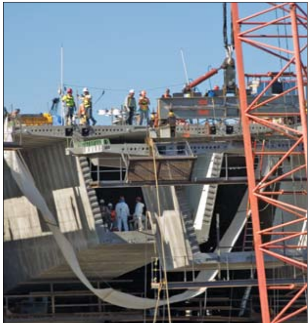
A close-up look of workers near the bridge segments.
