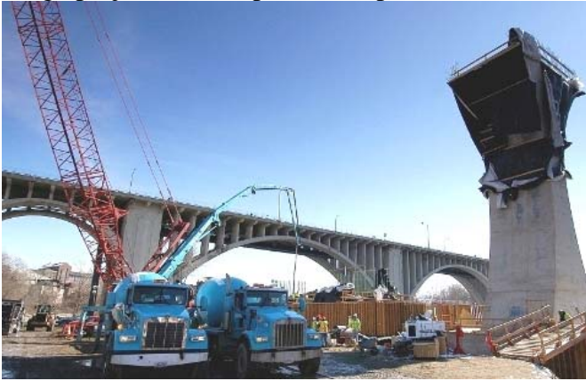
Cemstone’s Kenworth trucks at work on the I-35 bridge project.
