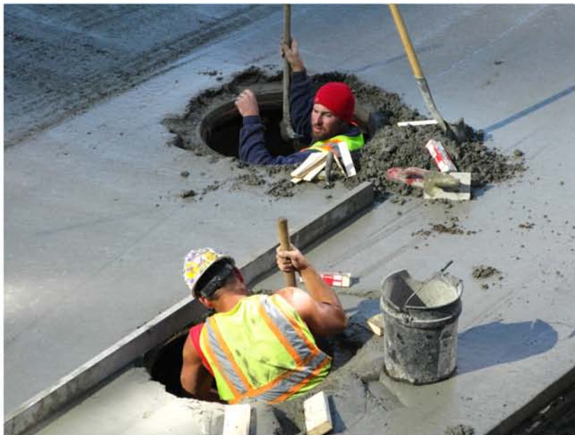
Crews placed 9 in. of new reinforced concrete pavement on top of the recycled material. The concrete mix consisted of a 0.4 water/cement ratio or lower, which reduced the cure time to two to three days.
